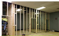
FUTURE TREATMENT ROOMS
